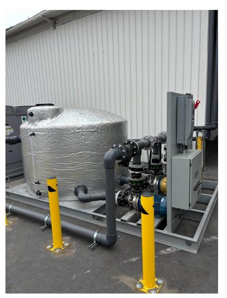
Additional equipment and infrastructure alongside the exterior for liquid nitrogen
